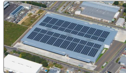
DPL Koriyama's roof-top solar panels generating 3.0MWp of energy per annum
